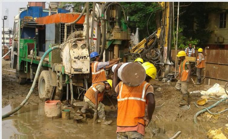
**DESTRUCTIVE DRILLING**, also known as DTH Drilling, is a method in which hammer blows are transmitted by the drill rods to the drill bit. It may be by wet percussion method, direct to hammer method or rotary method.
