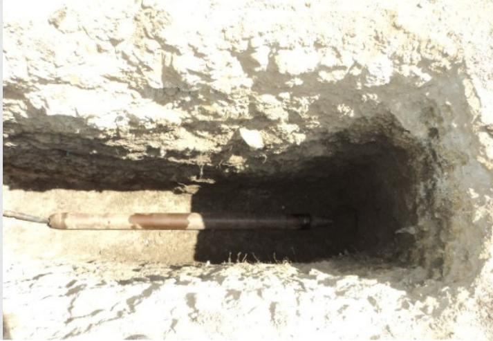
**PNEUMATIC MOLING** also known as Impact Moling, is a trenchless method used for pipe/cable laying. A self-propelled pneumatic hammer is used to drill through and cover short distances, without digging an actual trench.
