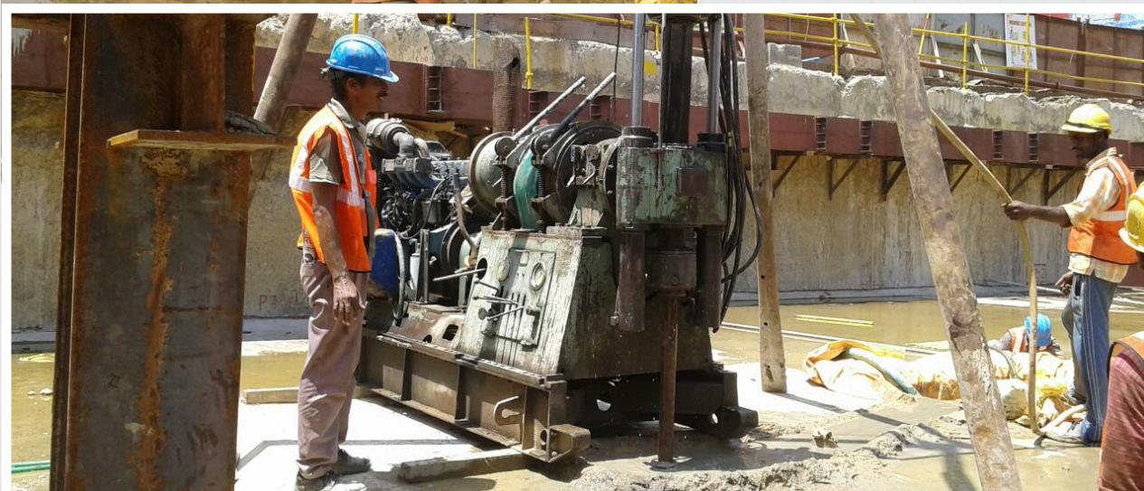
**RECHARGE WELL** is the exact opposite of a conventional well. It pushes the surface water back into the groundwater system.
