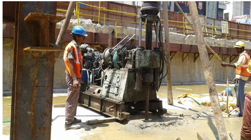
**GROUTING** is the process of injecting cement or relevant chemicals into the substrate, to fill voids. Grouting is used for soil stabilization, treatment of leakages inside tunnels and for strengthening soil bearing capacity. Different methods include Curtain Grouting, Consolidation Grouting, Permeation Grouting and TAM Grouting.
