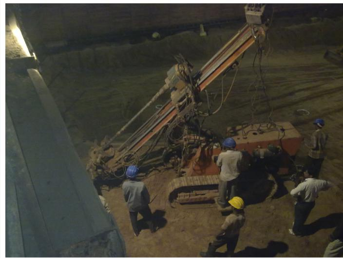
**GROUND ANCHOR** is a device that is designed to support structures and is used in geotechnical and construction applications. It can be referred to as a percussion driven earth anchor or mechanical anchor.
