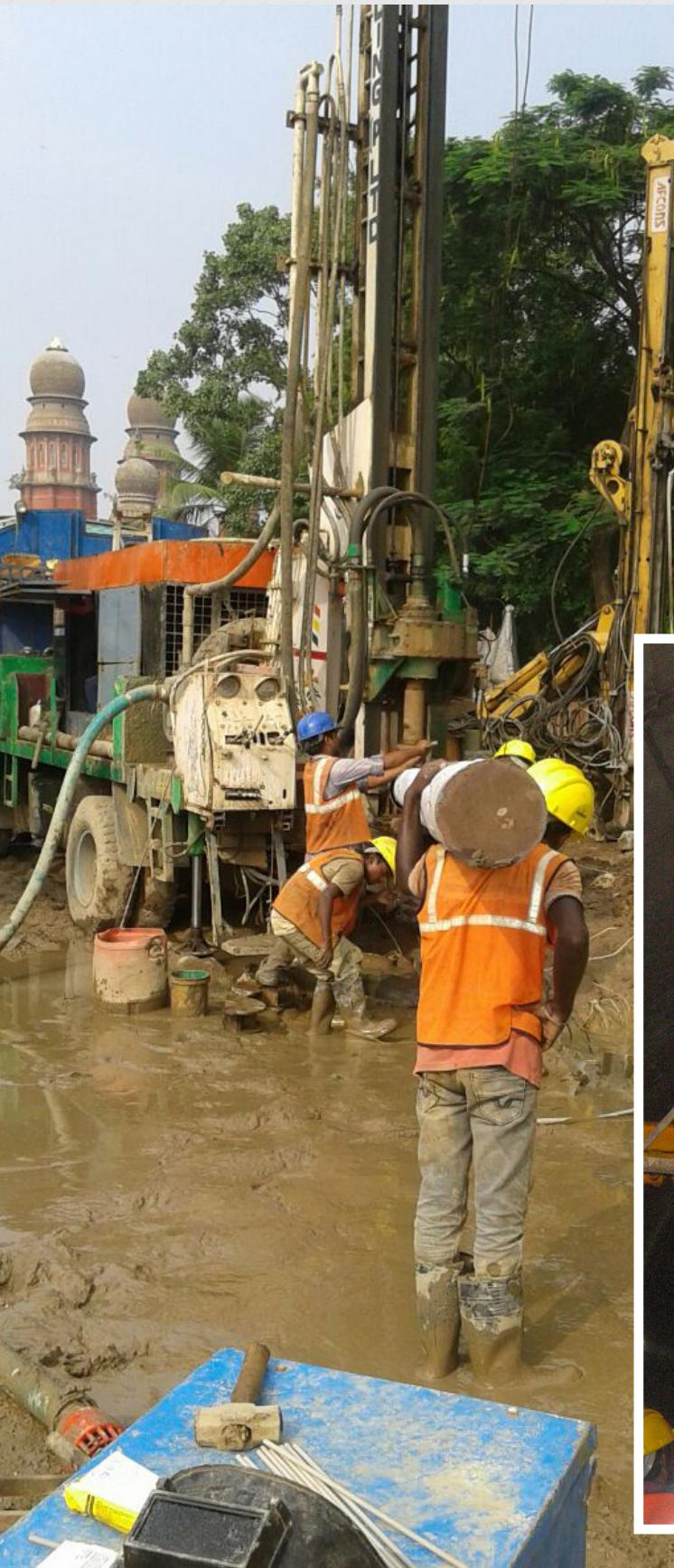
**DEWATERING** is a method of removal of groundwater or surface water from a riverbed, construction site, caisson, or mine shaft, by pumping. It is executed before subsurface excavation for foundations, shoring, or cellar space to lower the water table, and involves the use of submersible "dewatering" pumps, centrifugal pumps or application of vacuum to well points.
